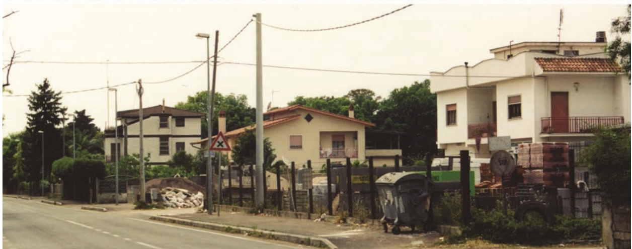
Figure 9 | The linear settlements along Via Laurentina (top picture) and along Via Ardeatina (bottom picture). In the first, commercial, artisan and industrial buildings prevail. In the central picture, the rural landscape located between the two linear settlements is shown. It is characterized by arable crops and by strips of riparian vegetation, growing along the ditches and at the foot of the steep slopes of tufaceous hills. Source: D. Cinti
