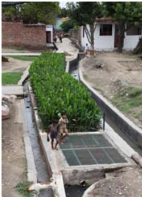
Figure 3. Completed Decentralised Wastewater Treatment System (DEWATS), Kachhpura settlement, July 2011.
