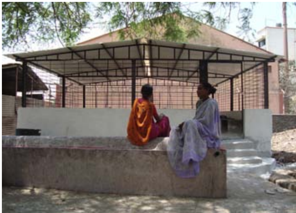
Figure 4. Completed classroom building at Tata Press quarry settlement, November 2009 [Source: Helena McDermott].
