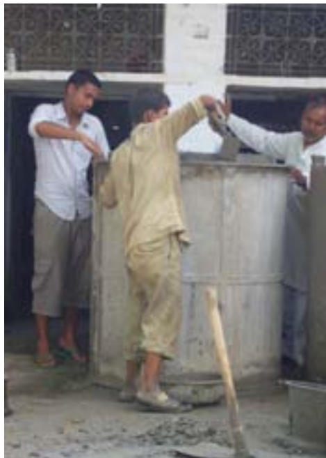
Figure 7. Student and contractors making a pre-cast concrete septic tank, Agra, July 2007.
