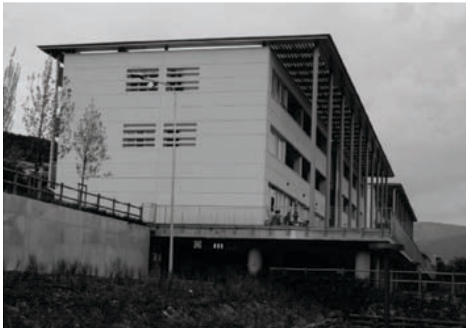
Figure 3. C.A.S.E. post-earthquake housing at Bazzano on the periphery of L’Aquila city (Alexander 2010: 335).
